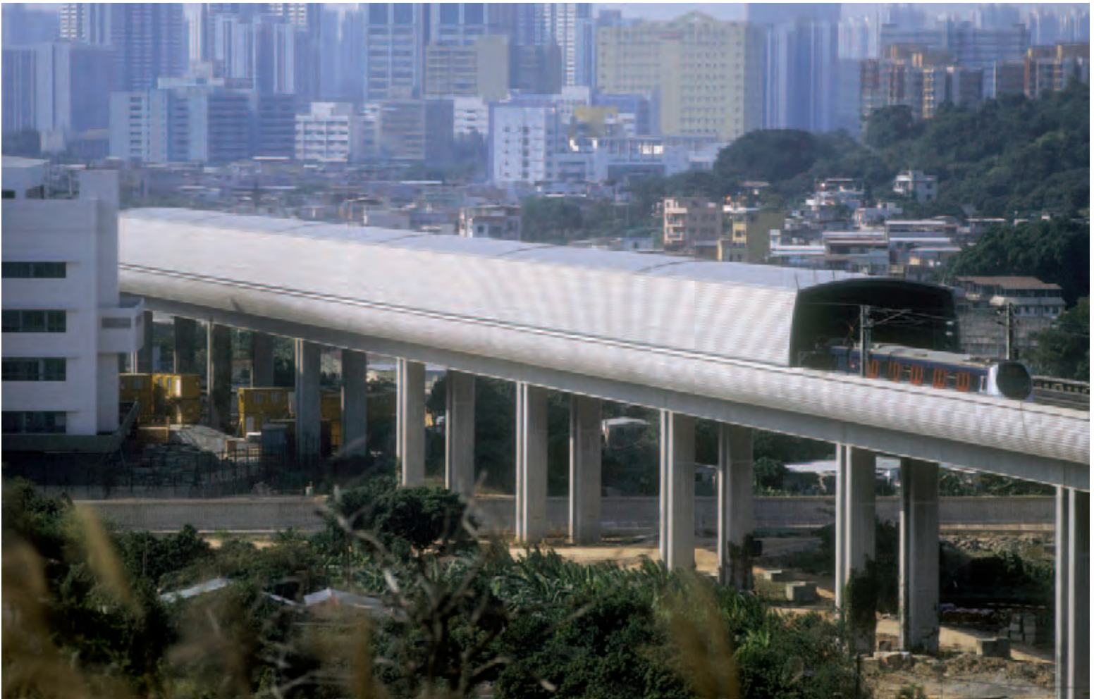
11. The full noise enclosure in use, adjacent to Pok Oi Hospital at Yuen Long.
