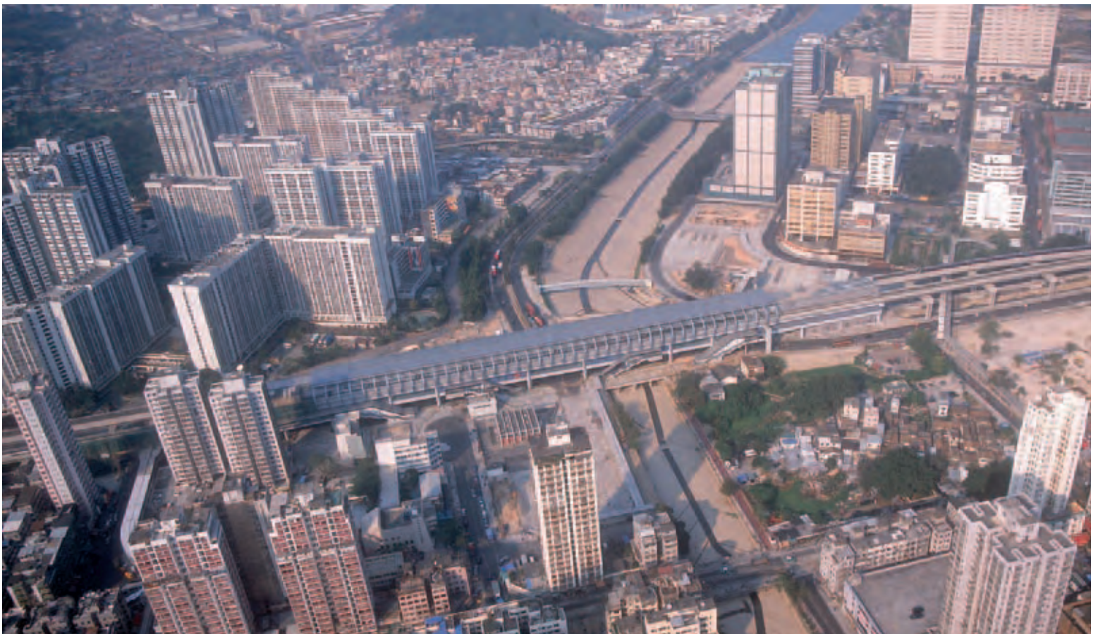
24. Long Ping station in context.
