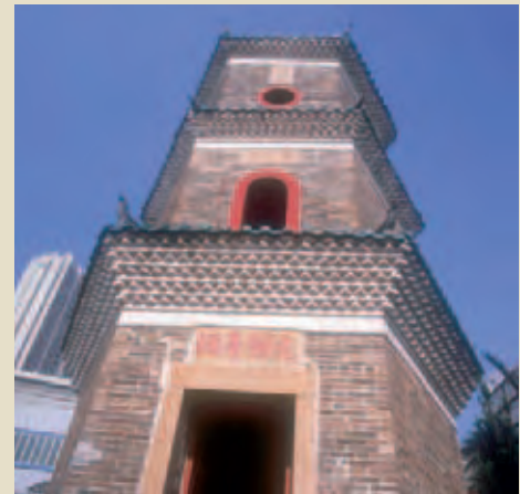
28. Tsui Shing Lau pagoda, showing ornamental brick corbelling.
