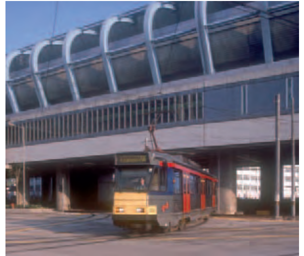
26. Tin Shui Wai station links to the existing LRT system.
