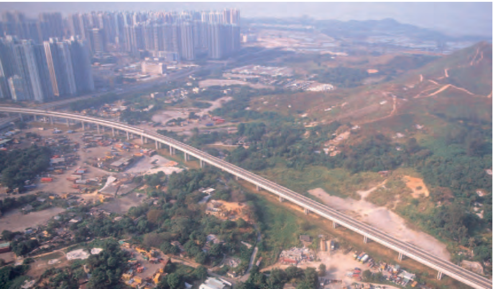
4. Yuen Long viaduct from the air, approaching Tin Shui Wai on the left.
