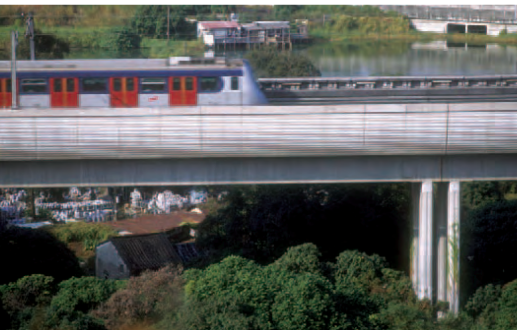
9. The parapet in use.
